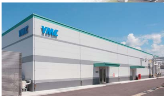
API Purification Plant
