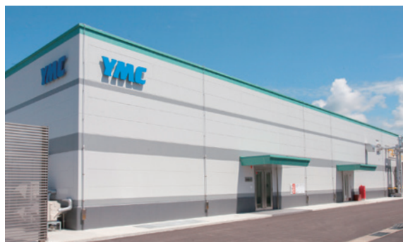
API Purification Plant
